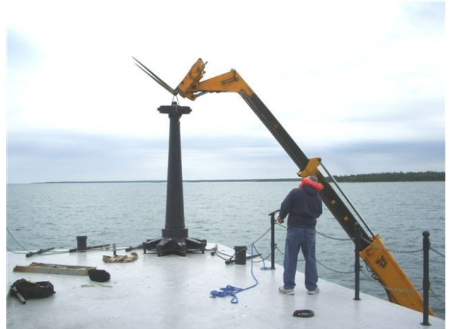
Removing the crane from the barge below.
