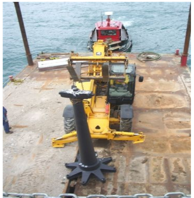
Special equipment on a barge below is used to remove the deck crane.
